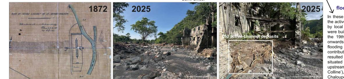
Fig. 10 - Destruction of 'Lazaret n°2', a historic building over 150 years old, by the active-channel widening of the Grande Chaloupe River during cyclone Garance
