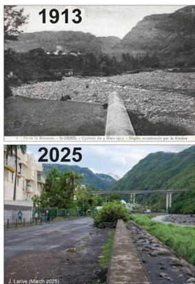
Fig. 11 - Breach in the Saint-Denis River dike, caused by the cyclone of March 4, 1913. Note that the area where the active channel was widened in 1913 has since been intensively built on
