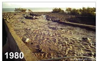
Fig. 13 - Breach of the "Patates à Durand" River dike during cyclone Hyacinthe
